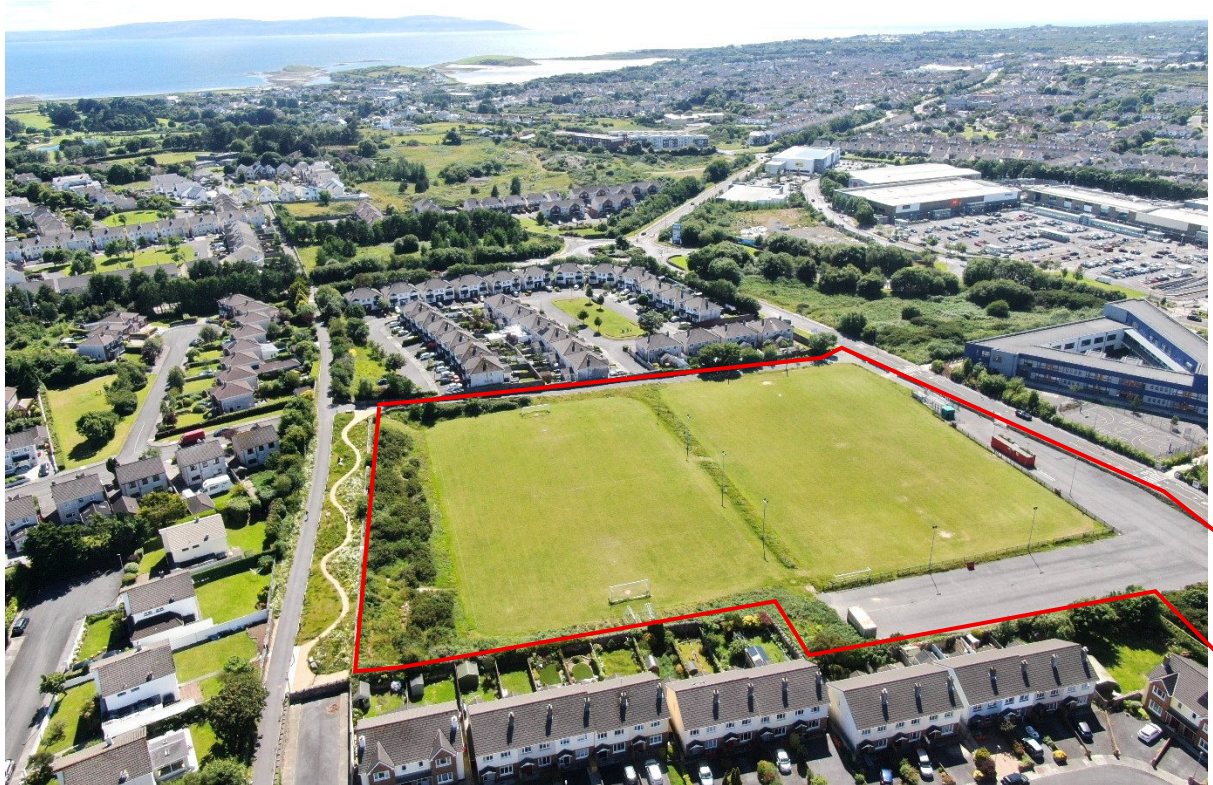
View 1: The Proposed Site in the foreground looking south back to Galway Bay. Gaelscoil Mhic Amhlaigh to the right and Gateway Shopping Park beyond.
